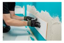
**6.** Fix wall tiles with Kiilto Superfix DF. Kiilto Flexfix or Kiilto Kerapid DF.
