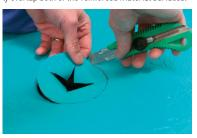
5. After the waterproofing membrane has dried, cut a round hole for the floor drain: ensure that the diameter of the hole is at least 40 mm smaller than the diameter of the floor drain, so that the rim of the Kerafiber layer stretches over the seal in the drain (follow the drain manufacturer's instructions). The thickness of the Kerafiber layer around the floor drain should be a minimum of 1.2 mm.
