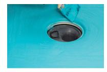
**13.** Fix the floor tiles with Kiilto Superfix DF, Kiilto Flexfix or Kiilto Kerapid DF. Attach the square cover centrally into the drain with tile adhesive. If there is still some waterproofing membrane visible between the drain and the cover, ensure protection by applying tile adhesive.
