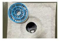
7. You can also seal the floor drain with a self-adherent Kiilto Easy Kaivolaippa reinforcement. Place Kiilto Easy Kaivolaippa on a dry, primed surface and press carefully into position. Cut a hole into it according to the drain manufacturer's instructions and press the tension ring into position.
