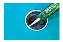
10. Seal the junction between the tension ring and the floor drain with Kiilto Pro Masa sealant. Kiilto Easy Kaivolaippa has been tested and approved in terms of its compatibility with the most common floor drain types.
