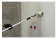
1. Ensure that the surface is dust-free and prime it using either Kiilto Keraprimer or Kiilto PrimerOne. Dilute the primer in accordance with the product-specific instructions. Allow the primer to dry for at least 30 to 60 minutes before beginning the waterproofing.
