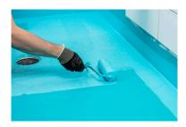
12. Roll a second coat of Kerafiber and allow to dry for 6-12 h/colour change before tiling. Check the thickness of the Kerafiber layer. Add Kerafiber on top of thin and/or porous spots and allow to dry properly. The total consumption of Kerafiber should be at least 0.8 l/m<sup>2</sup> and the layer thickness 0.5 mm.
