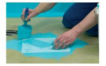
**4.** Apply waterproofing membrane around the floor drain (approx. 40 x 40 cm area), and turn the prepared floordrain patch over the drain. When using a separate sealing flange, contact our technical support or consult your drain supplier for instructions.
