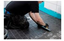
14. Apply Kiilto Pro Floor tile grout with a squeegee. Press the product firmly into each joint, ensuring that they are completely filled with the product. Wash off excess grout with a sponge 15 to 30 minutes after application. To ensure that the colour of the seams remains uniform, sponge should only be minimally moist. The seams between tiles can be shaped using a thick electrical wire.
