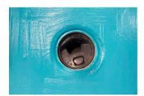
**9.** Apply Kiilto Kerafiber on the reinforcement sheets on all sides of Kiilto Easy kaivolaippa. Apply Kerafiber to the entire area.
