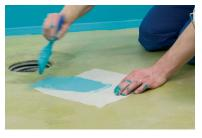
3. The floor drain can be waterproofed with two Kilto Lattiakaivovahvike floordrain patches. Place one floor drain patch on the floor and brush Kerafiber over it. Place the other patch over the first patch crosswise and brush Kerafiber over it
