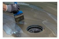
1. Ensure that the surface is dust-free and and prime it using either Kiilto Keraprimer or Kiilto PrimerOne. Dilute the primer in accordance with the product-specific instructions. Allow the primer to dry for at least 30 to 60 minutes before beginning the waterproofing work.
