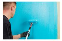
**4.** Use a roller to apply Kerafiber over the entire wall surface and allow the product to dry for at least 2 hours or until the colour changes.
