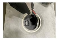
8. Make sure that the tension ring is properly seated and cut off the edge of reinforcement sheet protruding from underneath.
