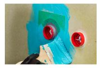
3. When reinforcing pipe channels, you may opt to use either prefabricated reinforcement pieces or pieces of Kiilto Nurkkavahvike corner reinforcement tape. Install the reinforcement pieces onto wet Kerafiber and brush Kerafiber over it to ensure wetting. Ensure that each piece is thoroughly saturated by brushing them with waterproofing agent. Channels can also be sealed using Kiilto Pro XPU Adhesive and reinforcement sealant before they are waterproofed.
