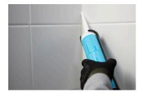
15. Remove any excess grout in the corners. Seal corners and channels or penetrations with Kiilto Pro Sanitary silicone or Kiilto Pro Silicone E. The wet room is ready for use on the following day. However, any heating elements in the floor can only be used a full week after the seams have been finished.
