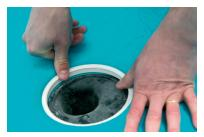
Press a suitable tension ring into position. Cut off any excess Kerafiber under the ring.
