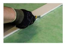
1. Before you start, cut the required number of KerSafe + foils ready for the job. If you need more open time for the foil installation, prime the substrate. Mix liquid A and powder X components of the adhesive carefully. The pot life of a mixed product is min. 1 h and coverage approx. 12 m<sup>2</sup>.
